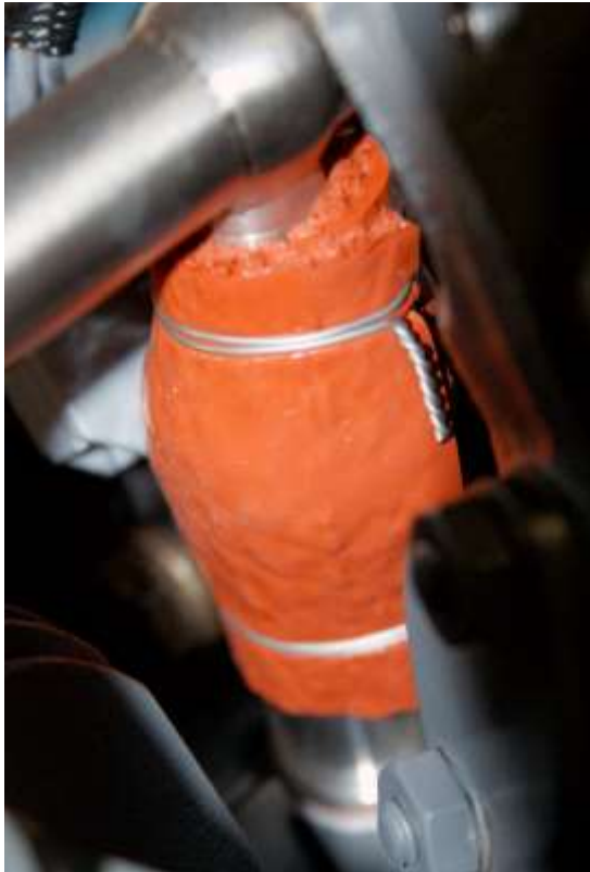
Figure 10 Installed Fire Sleeve P/N 01M29868
